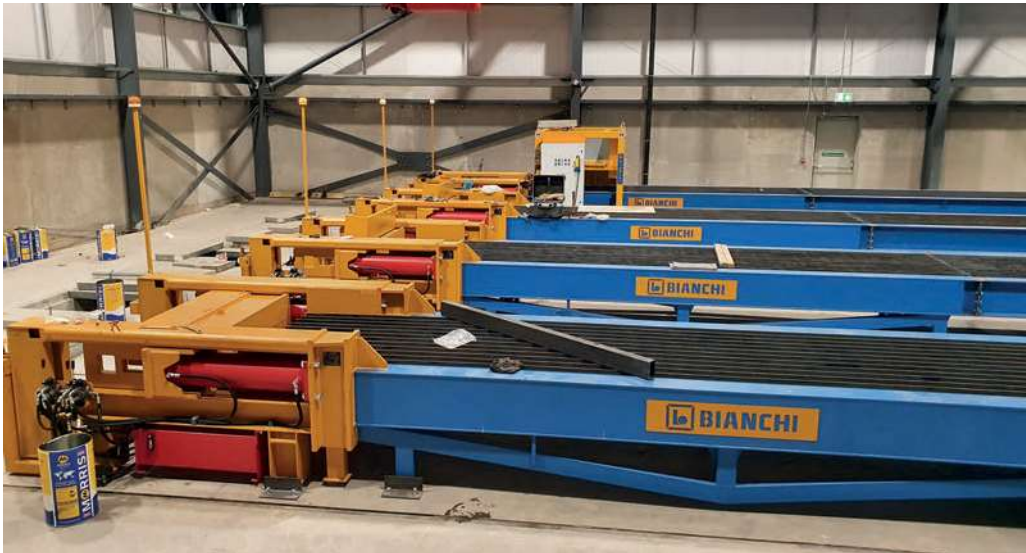
The first four moulds installed
