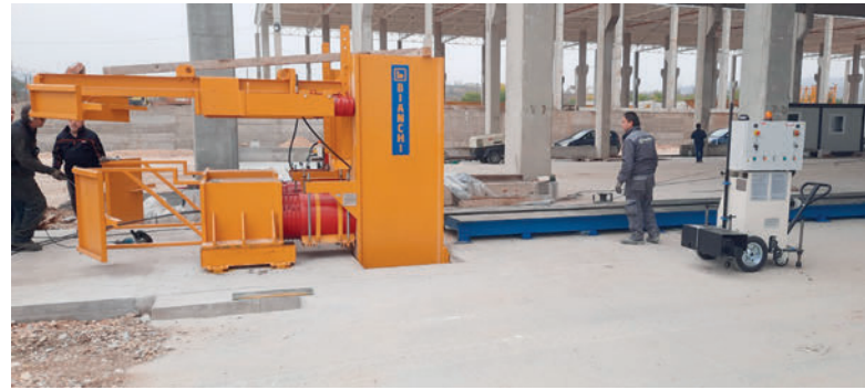
Strands anchoring structure
