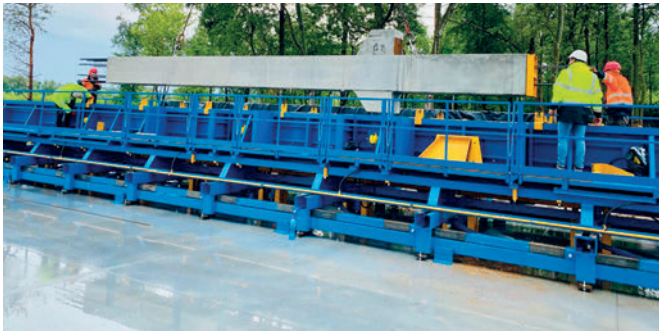
Precast concrete Column
