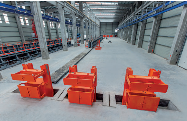
Site for beam production
