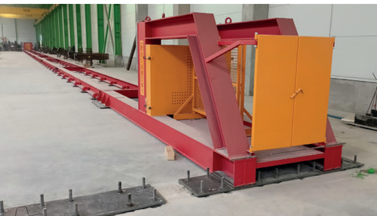
First line installed
