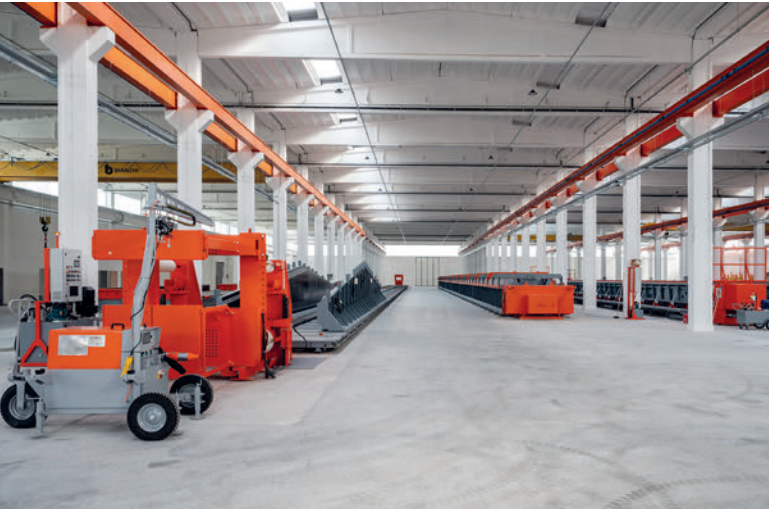
General view of formwork, beam track and wing formwork
