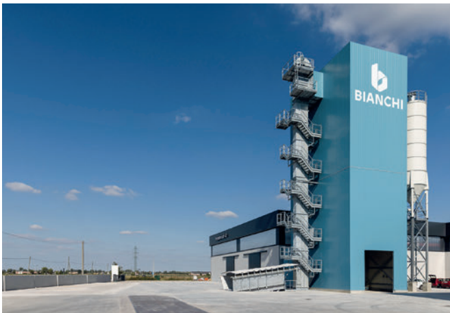
Exterior view Bianchi Prefabbricati
